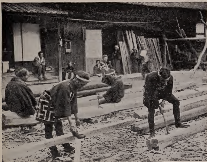
CARPENTERS AT WORK
